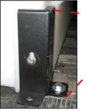
Figure 2-5. Drill Only 1 Hole for Corner Bracket
