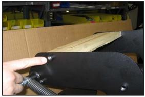
Figure 2-30. Remove 2 Screws Securing Wood Brace
